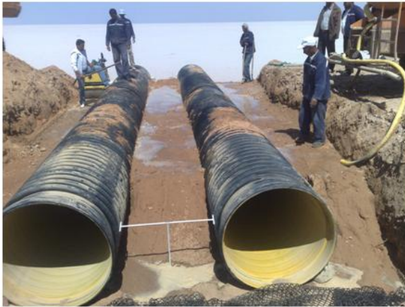
Figure 9: PEHD reinforced tubes installation.
