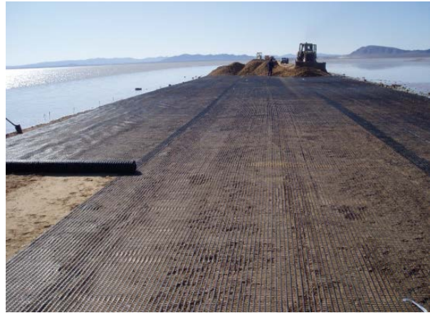
Figure 8: Laying the biaxial geogrid over the first lift of the embankment
