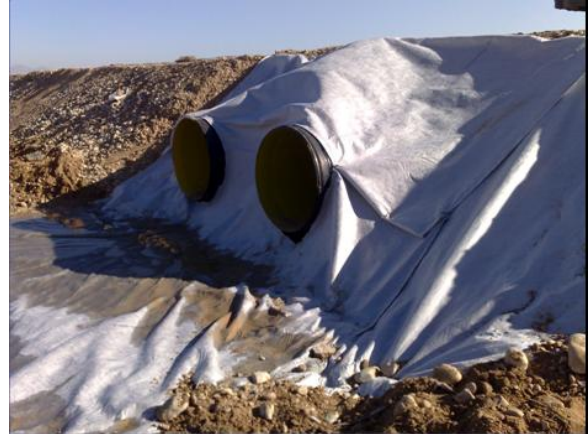
Figure 10: PEHD tubes extremity protection.
