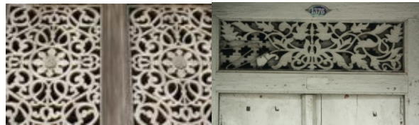
Fig. 7. Tebuk tembus to facilitate ventilation.
