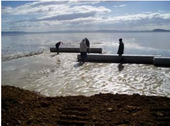
Figure 7: Laying directly over sabkha surface a nonwoven geotextile GT 1
